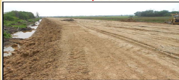
Fill Embankment & compact El.+3.90m.
