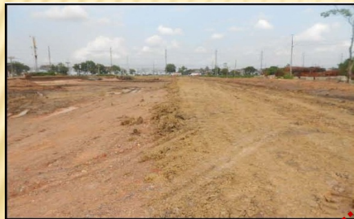
Fill Embankment & compact El.+3.70 m.
