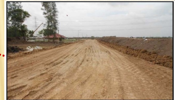
Fill Embankment & compact El.+2+50m.
