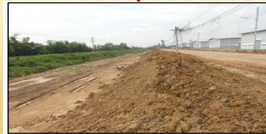
Fill Embankment and compaction El.+4.30 m.
